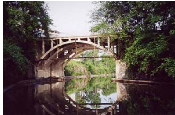
Troost Bridge as it is today - before construction began.
